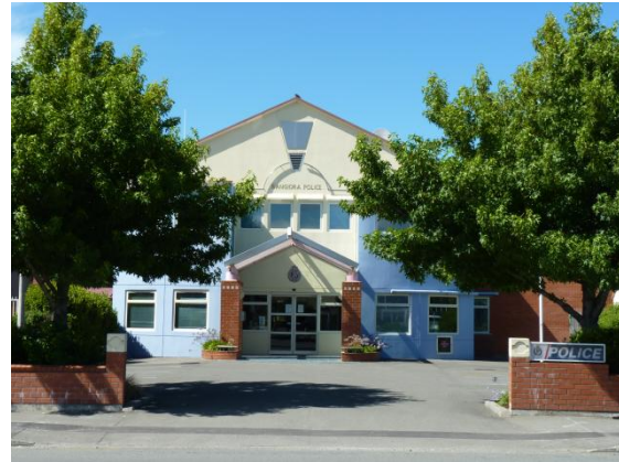
Rangiora Police Station
